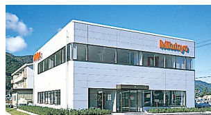
Suwa Sales Office
