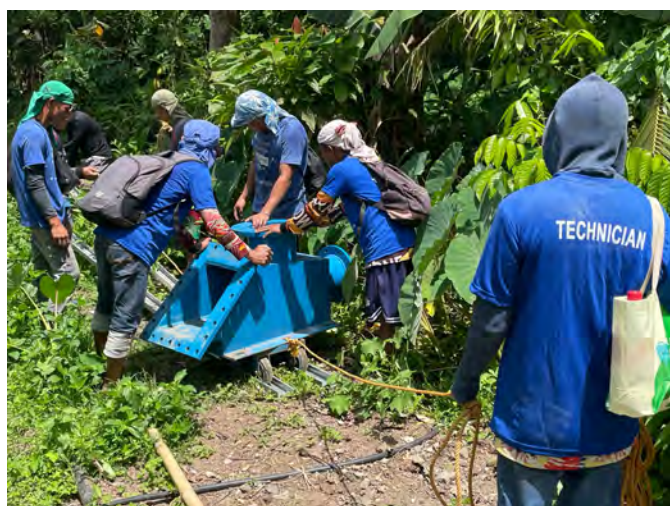
AIDFI Technical Services Personnel transporting the 8" ram body down to the source for installation
