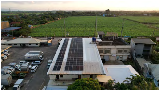
AIDFI office and workshop roof with 77 solar panels
