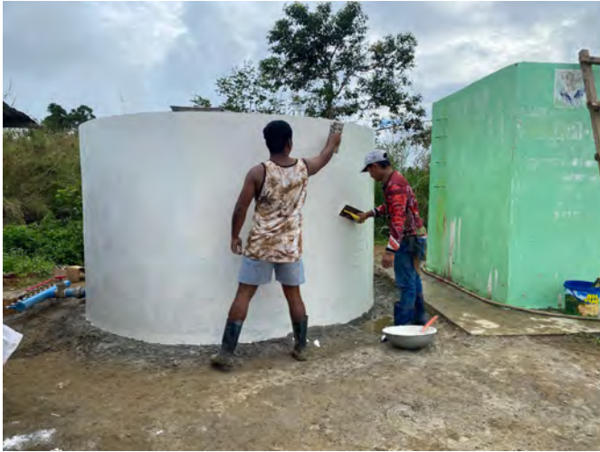
Team working on the reservoir in Tamac project
