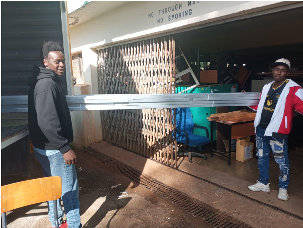
Photo 6.2-4: Arrival and on-site storage of inverters, electrical components, and mounting structures prior to installation.
