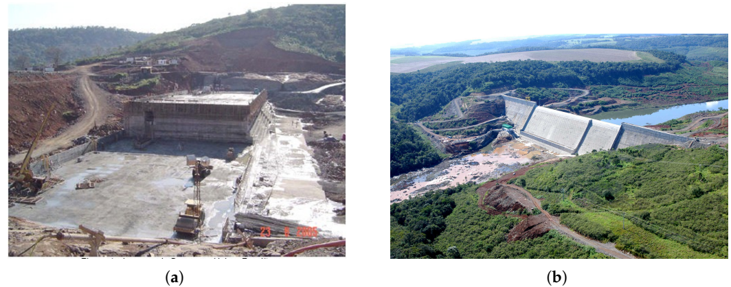
Figure 1. Pictures of the Fundão dam: (a) Under construction, (b) after construction [42].
