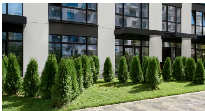
Стилобат Wellton Towers
