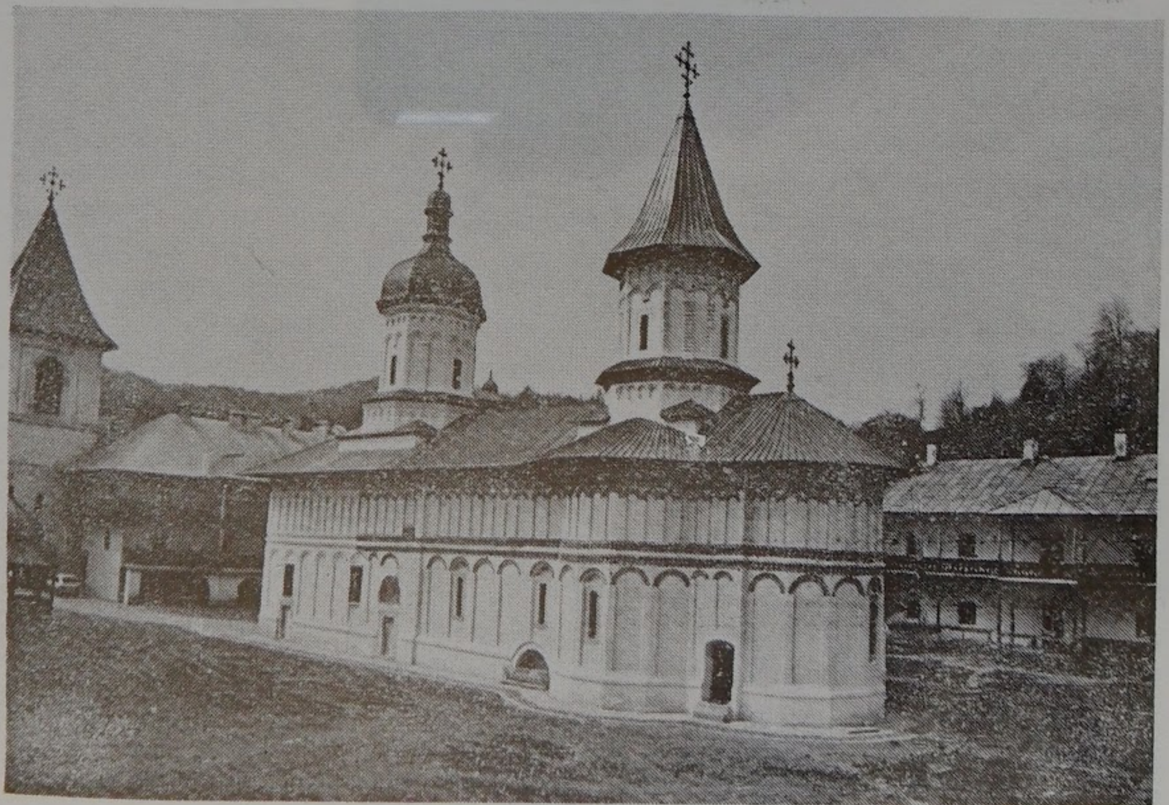
Inside view of the main church in the courtyard of the Monastery of Sekoul
