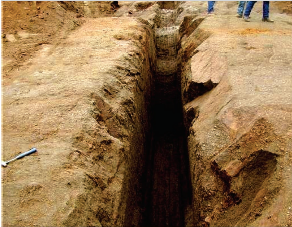
Fig. 9. Moderately Weathered Bedrock Foundation and Seepage Cutoff Key
