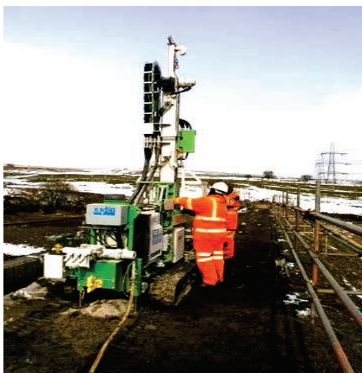
Fig. 4. Tube-a-manchette grouting works
