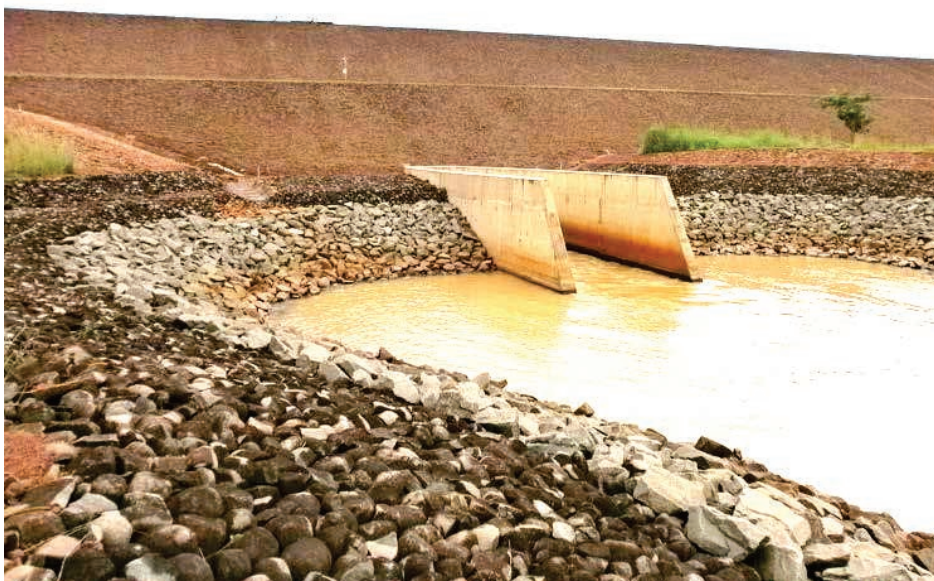
Fig. 7. Downstream face of dam
