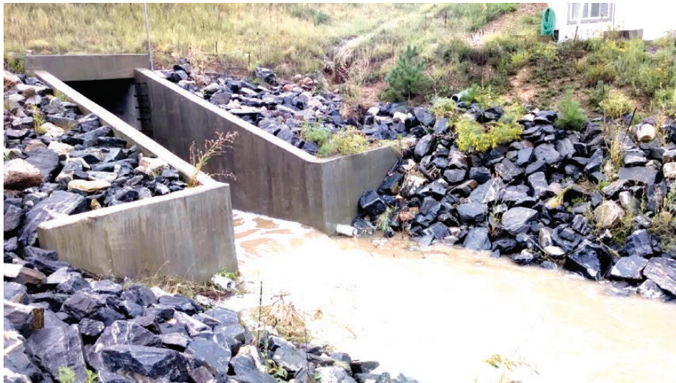
Fig. 8. Service Spillway Stilling Basin During Operation in 2013
