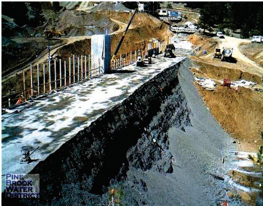
Fig. 5. Downstream Face During RCC Structure Construction
