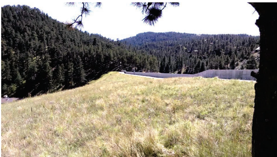
Fig. 6. Downstream Dam Slope with Grass Vegetation - Post Construction
