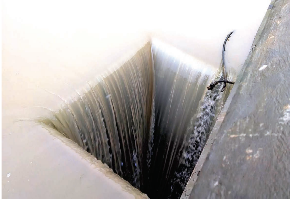
Fig. 7. Service Spillway Crest During Operation in 2013
