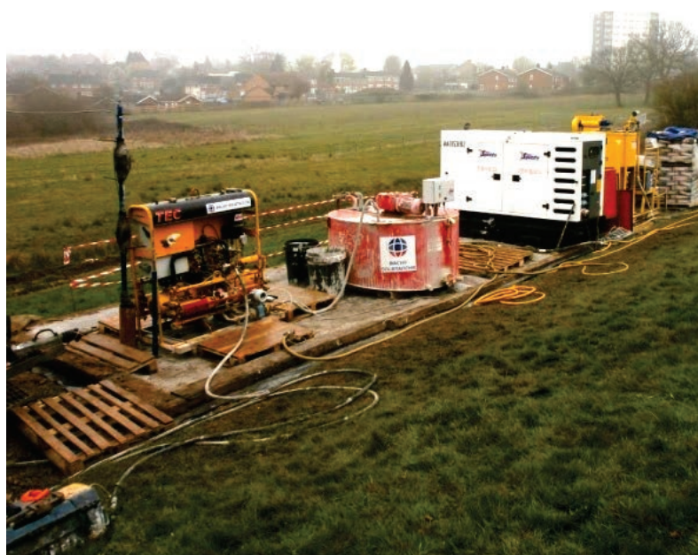
Fig. 6. Drilling & grouting plant
