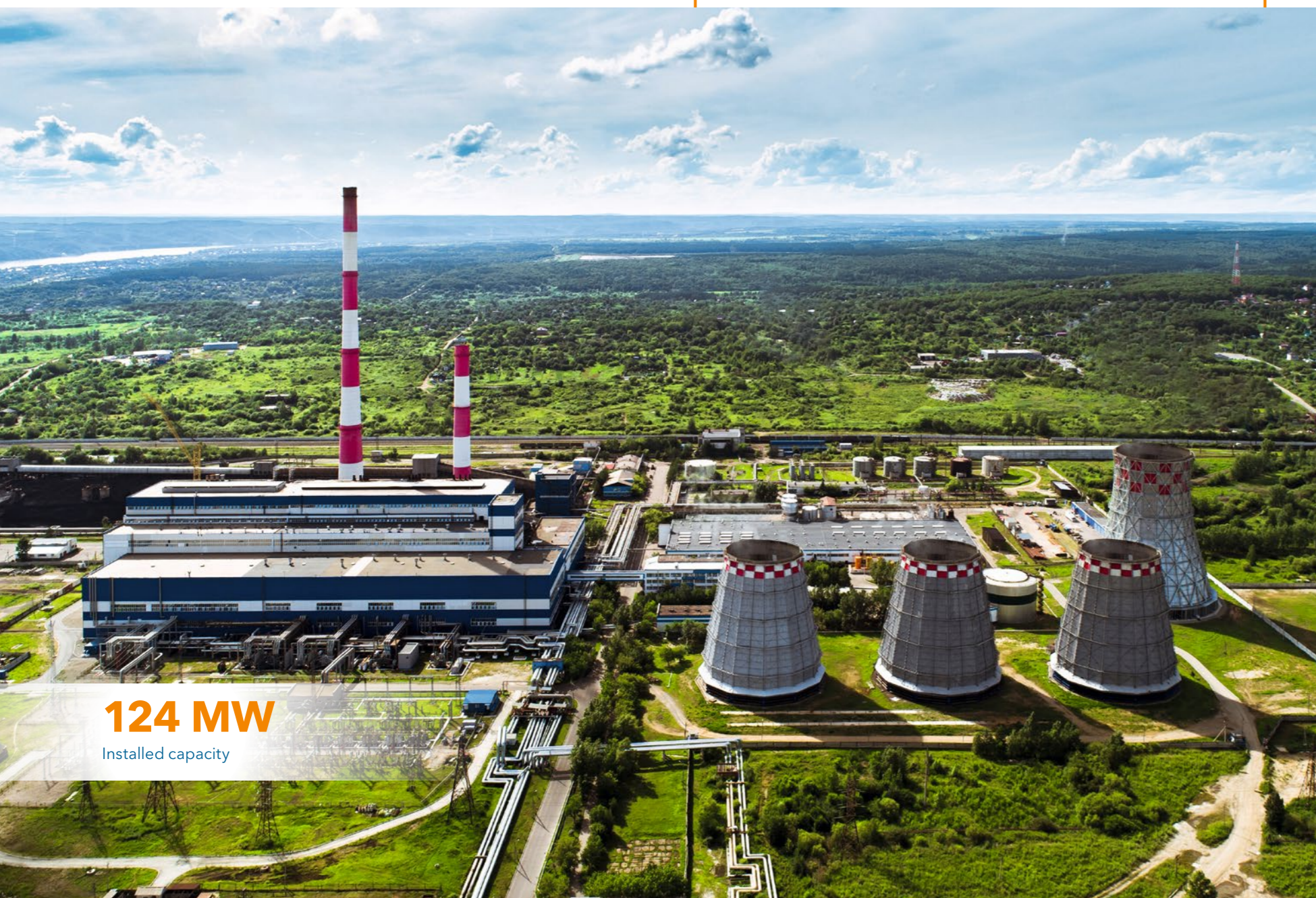
Blagoveshenskaya CHPP in Amur Region, second stage
